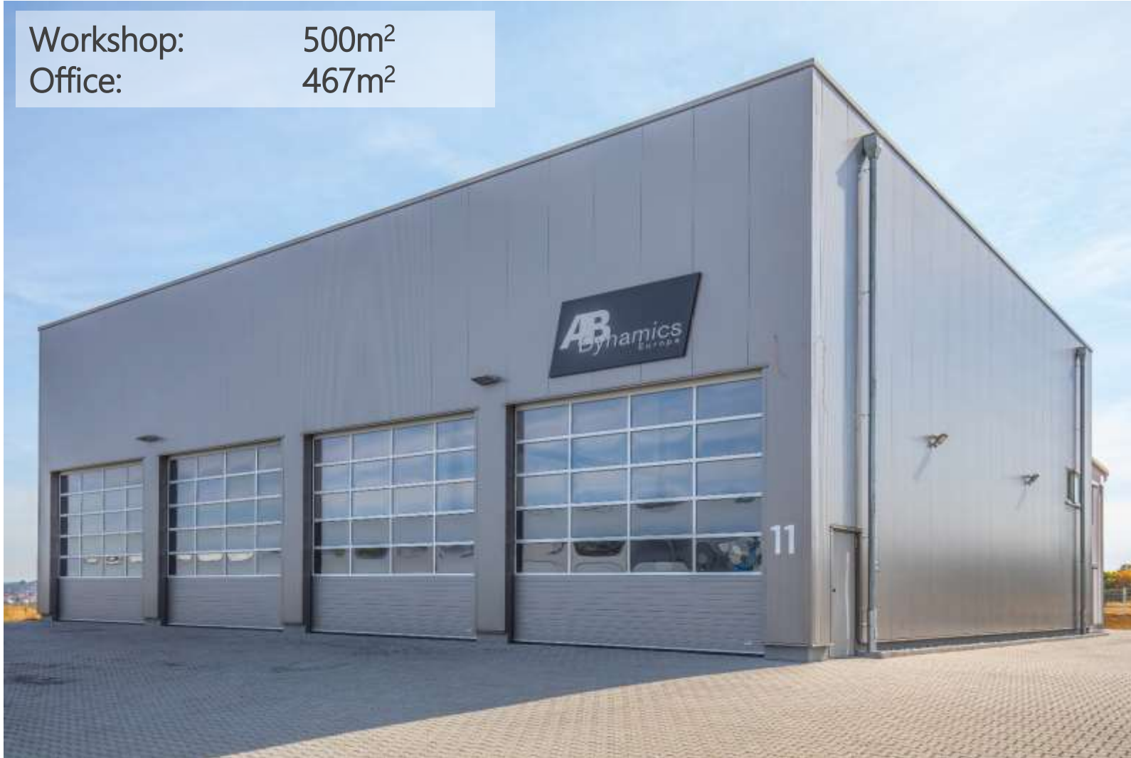
External view (September 2018)
